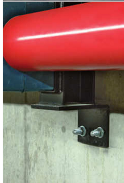
Apply recommended fastening torque with a calibrated torque-wrench
