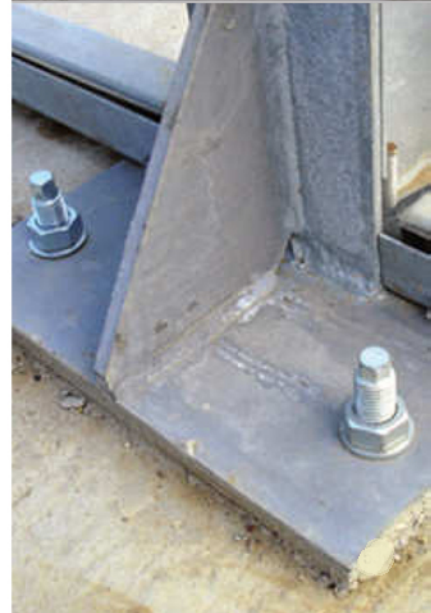
After the specified cure time, install the fixture and apply the recommended fastening torque with a calibrated torque-wrench
